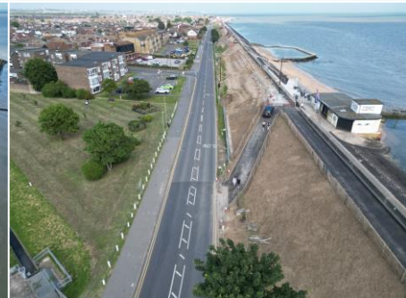
Concord Café access ramp and embankment
