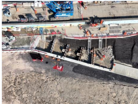
Concord Beach – new access jetty ramp and concrete apron slabs
