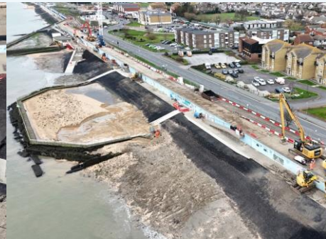
Concord Beach revetment approaching completion
