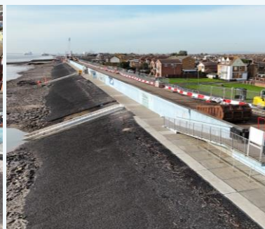
Revetment and new step looking west along the shoreline
