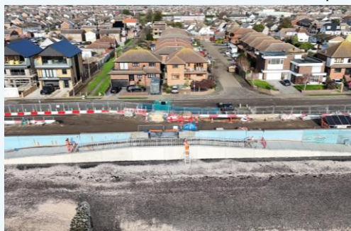
Chapman Sands ramp construction
