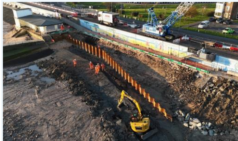
Steel sheet pile wall – Concord Beach
