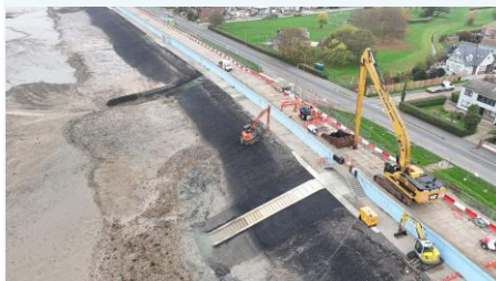
Precast steps at Eastern Esplanade
