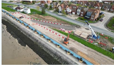
Temporary works at Thorney Bay, photograph courtesy of Hesselberg Hydro
