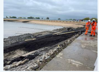
Installation of the new revetment
